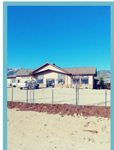
Our Completed New Addition!
